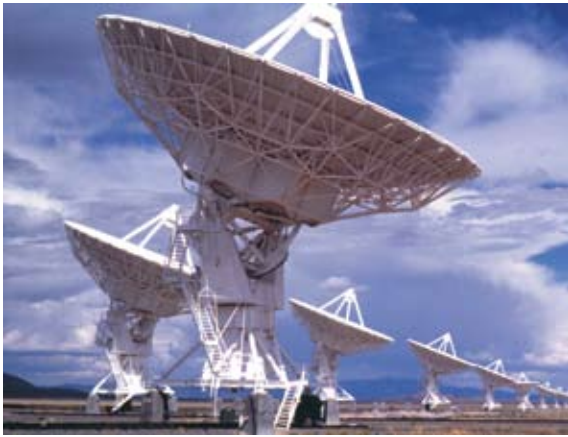
The Very Large Array, near Socorro, New Mexico, consists of 27 radio antennas in a Y-shaped configuration.
